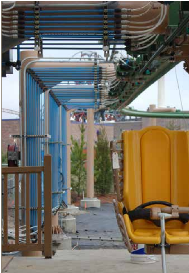
Screw type beam clamps
